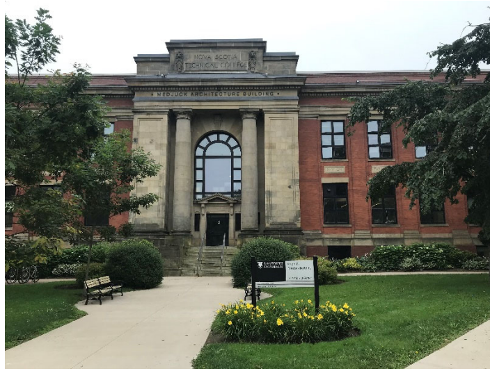
Main entrance Building H
