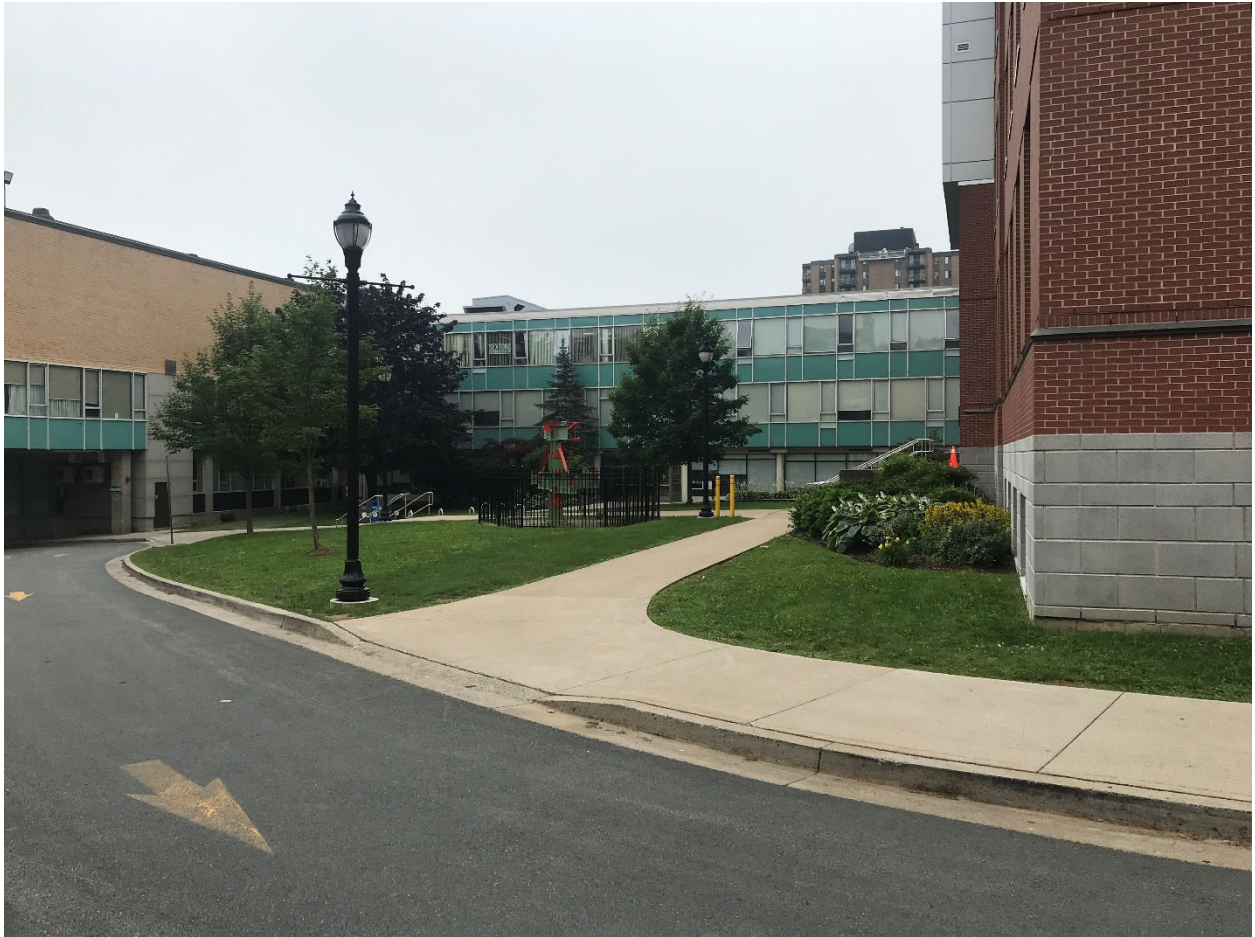
Building B as seen from near the H Building
